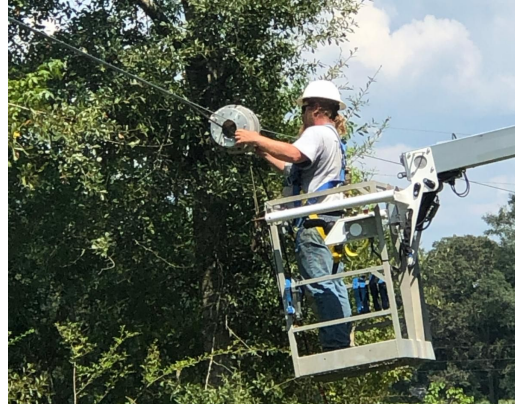
Contractors string fiber in Richton for the Brewer substation pilot project.
